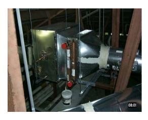
Building 631 Test: DOAS system consisted of replacing existing attic-mounted makeup air units with a new exterior custom air handler unit (AHU), tied into existing 4 pipe system, to provide deep dehumidification of outdoor air with a DX evaporator coil downstream of a chilled water coil.
